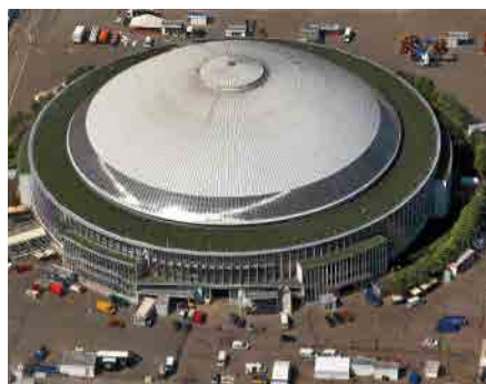
Pavilion "Z" has a diameter of over 120 m, the dome is 46 m high
